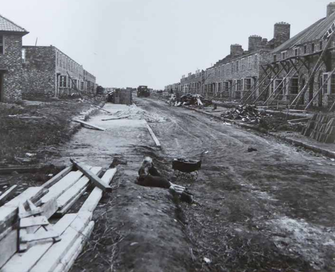
Norris Green takes shape: roofs are added to this road off Broad Lane, July 1926. Image courtesy of Liverpool Records Office.
